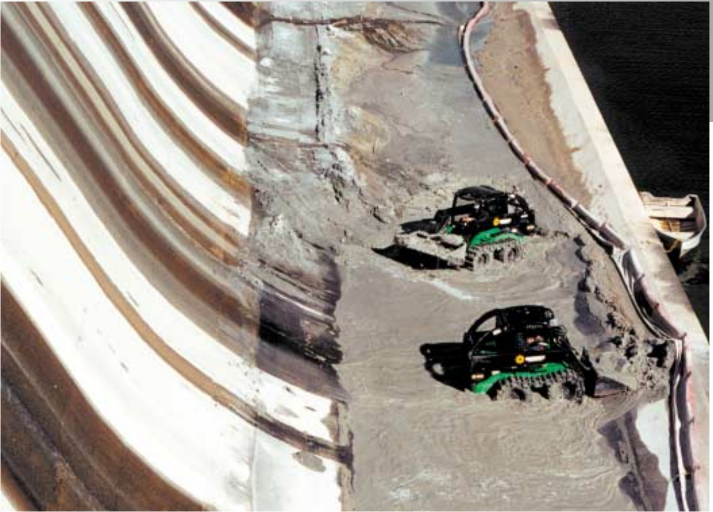
Two skid-steer loaders removing silt from the spillway of a dam in North Carolina
