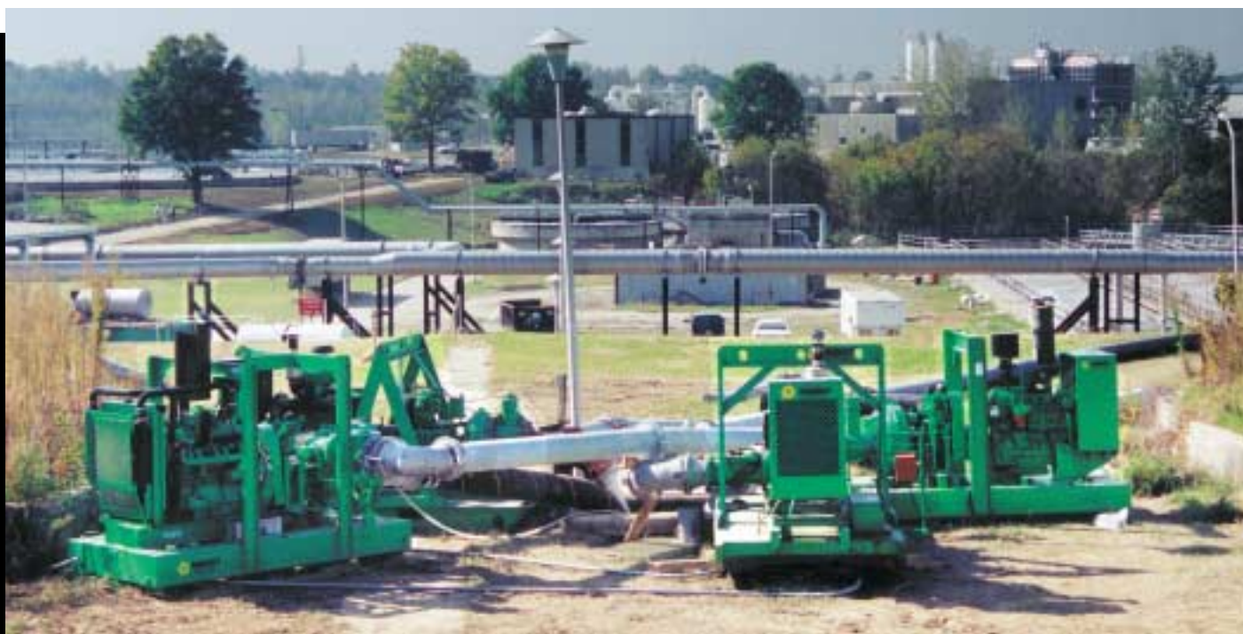
Four large diesel-driven trash pumps acting as a sewer bypass near Charlotte, North Carolina
