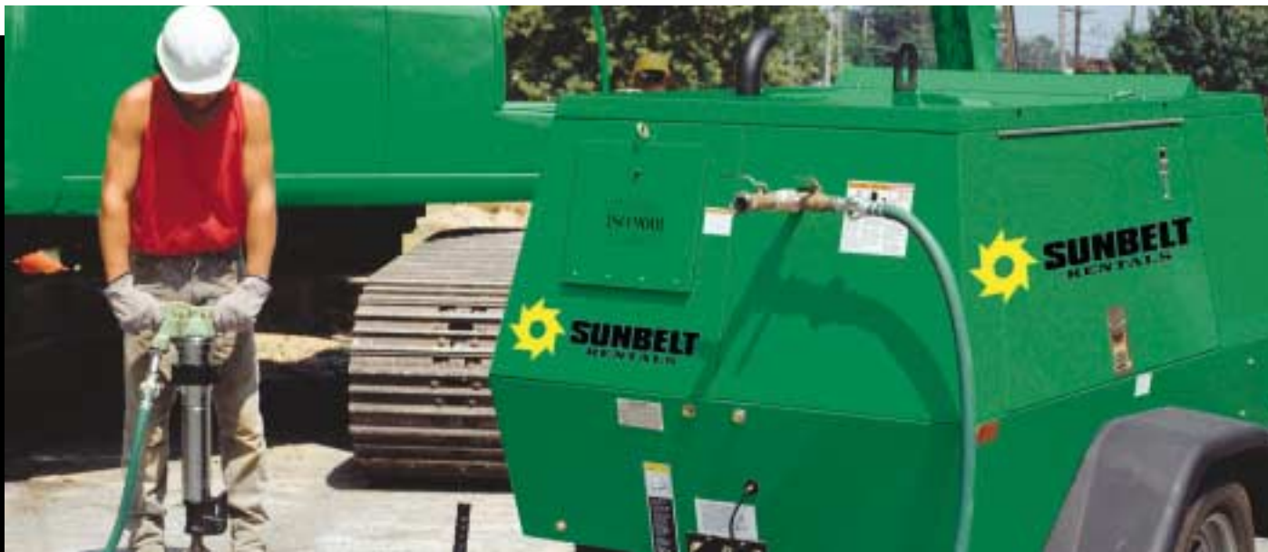
A portable diesel air compressor and pneumatic demolition tool
